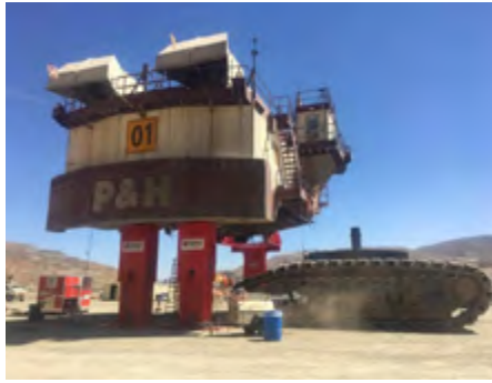
Pakka Jacks lifting stage.
